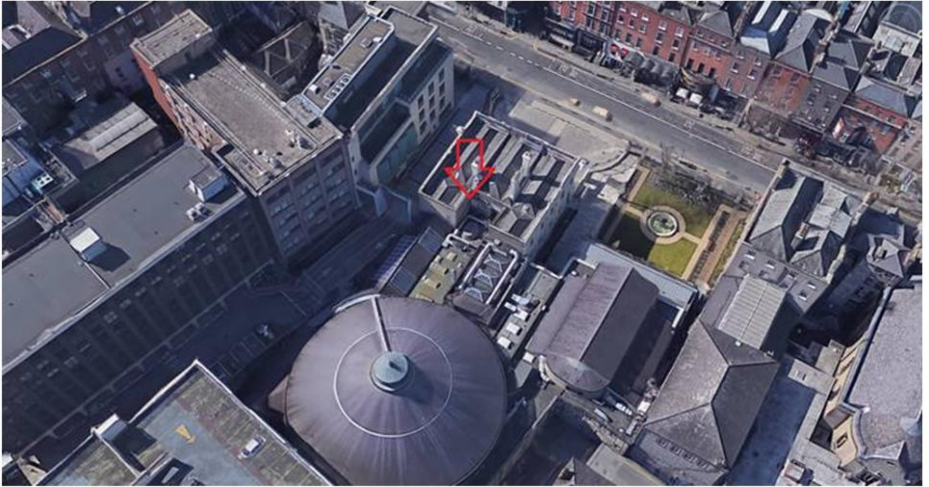
Image: Ariel View from South, red arrow indicates location of proposed single door opening to existing fire escape route across first floor roof
